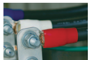
Wiring of lead wires
