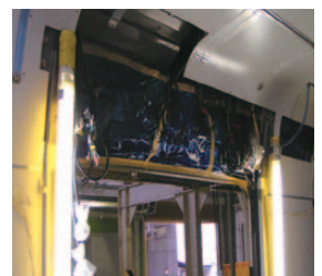
Wiring in a railway vehicle
