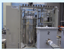
6.6kV 200A class FCL system
