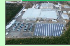
Solar power at the copper foil plant
