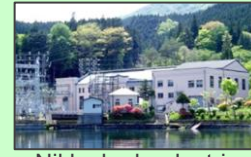
Nikko hydroelectric power station
