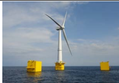
Fukushima floating offshore wind farm demonstration research
