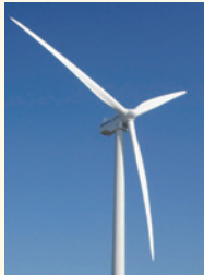
Cables for wind power generation
