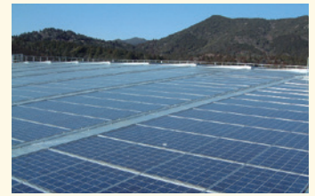
Cables for solar power generation
