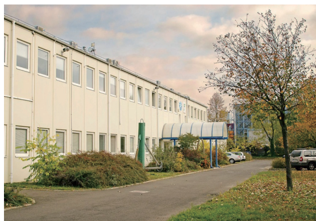
Figure 1 The building of FETI in Budapest, Hungary where all the offices and laboratories are located.
