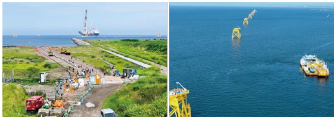
Cable laying during the Ishikari Bay New Port offshore wind power project
