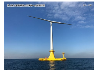
Status of installation of floating offshore wind power in an actual sea location
