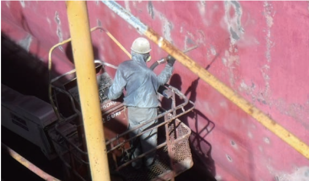
Figure 9 Sand blasting operation.
