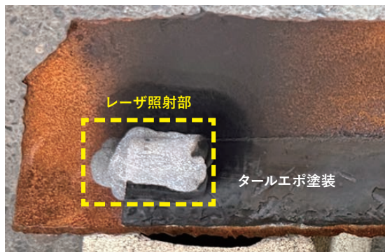
図15 沿岸地域で錆びた鋼材と上部に塗布されたタールエポ塗料の除去事例 Case study: Removal of rusted steel and tar-epoxy coating applied to the surface in coastal areas.
