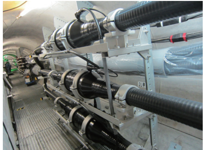
Figure 3 View of CSJ in Suruga Higashi-Shimizu Second Line.
